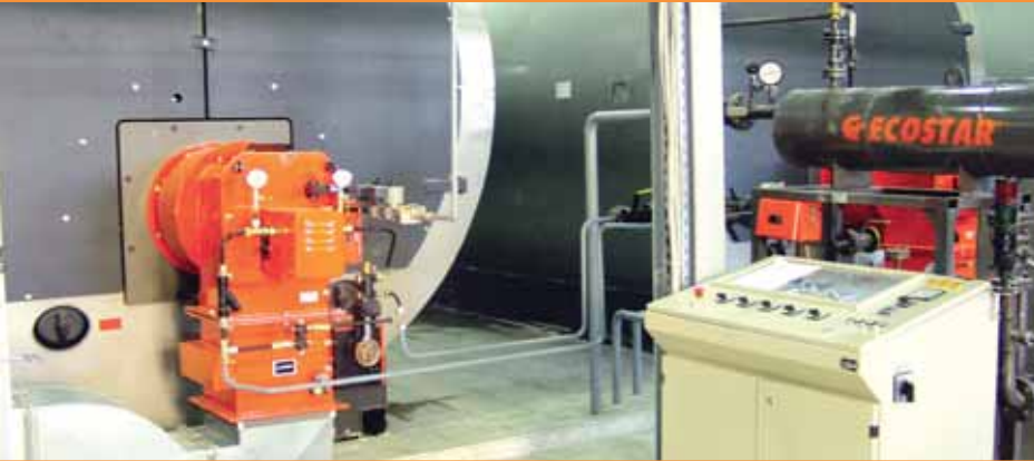
Motorin Pompalama Grubu Light Oil Pumping Station
